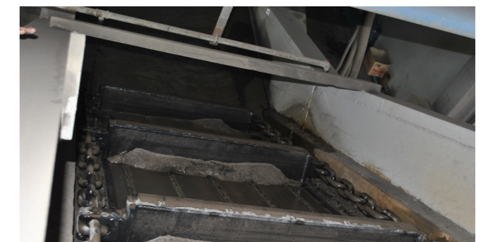
Image 19. O Series Ash Handling Chain
